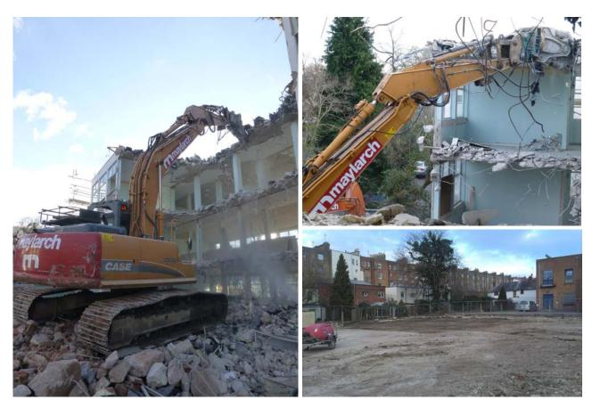
Demolition and asbestos removal of a 3 story reinforced concrete framed building in a highly sensitive residential area.
