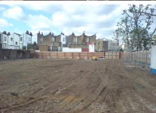
This was the first stage of a large regeneration scheme that consisted of the demolition of 36 town houses, ancillary buildings, hard and soft landscaping and arboriculture works. Maylarch were tasked with supplying all temporary service supplies, welfare facilities and site supervision. An asbestos survey was carried out prior to Maylarch getting involved in the project.
